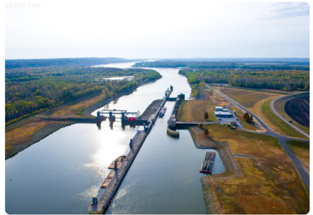
Aerial view of Jerry F. Costello Lock and Dam near the mouth of the Kaskaskia River in Randolph County.
