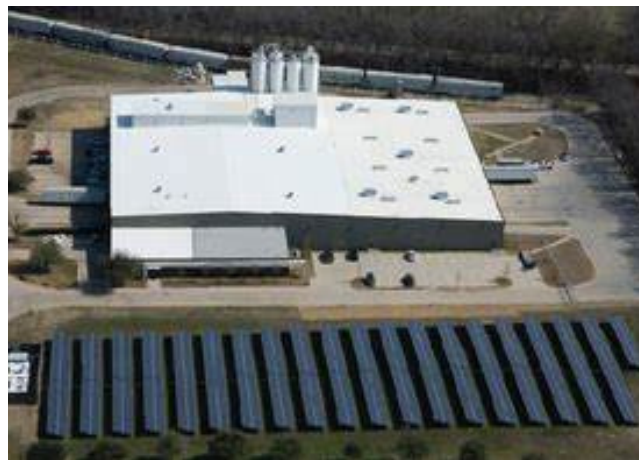
Manner Polymers' new PVC compounding plant in Mt. Vernon will have a 15-acre solar farm.
